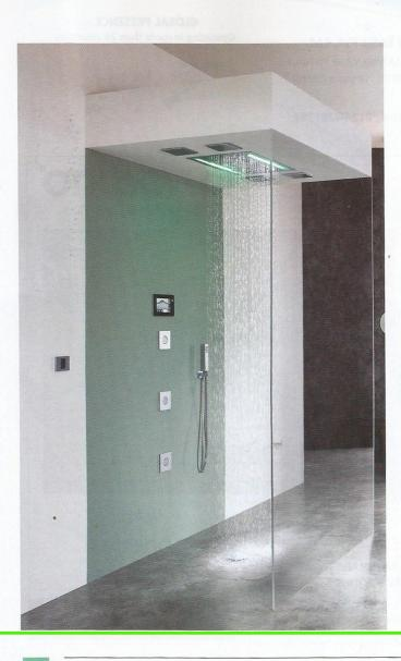
RAFF has developed and applied the touch-screen technology to a multifunction shower system, with the aim of making the use of a highly engineered product easy for the consumer. By adopting a technology already familiar to smartphones and tablet users, the shower touchpad allows control of several multimedia functions with a simple hand touch. After an intense research and development process, the final products have been able to meet all expectations in terms of design and functionality.
